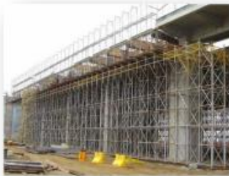
Scaffolding with Inspection
